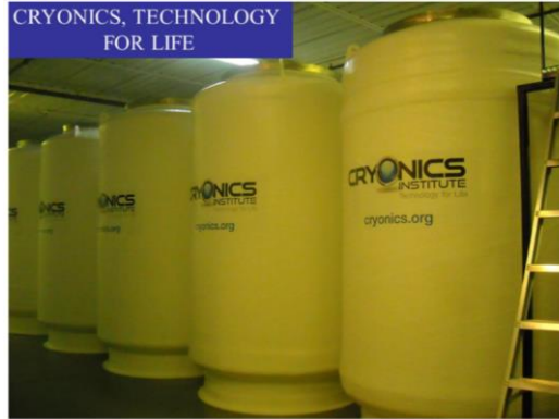
Figure 2: Storage area where large cryostats containing liquid nitrogen (LN) are kept in which the patients (typically 6 per unit) are stored in LN at -196 degrees. The logo on these thermos reads, “Cryonics, technology for life.”
